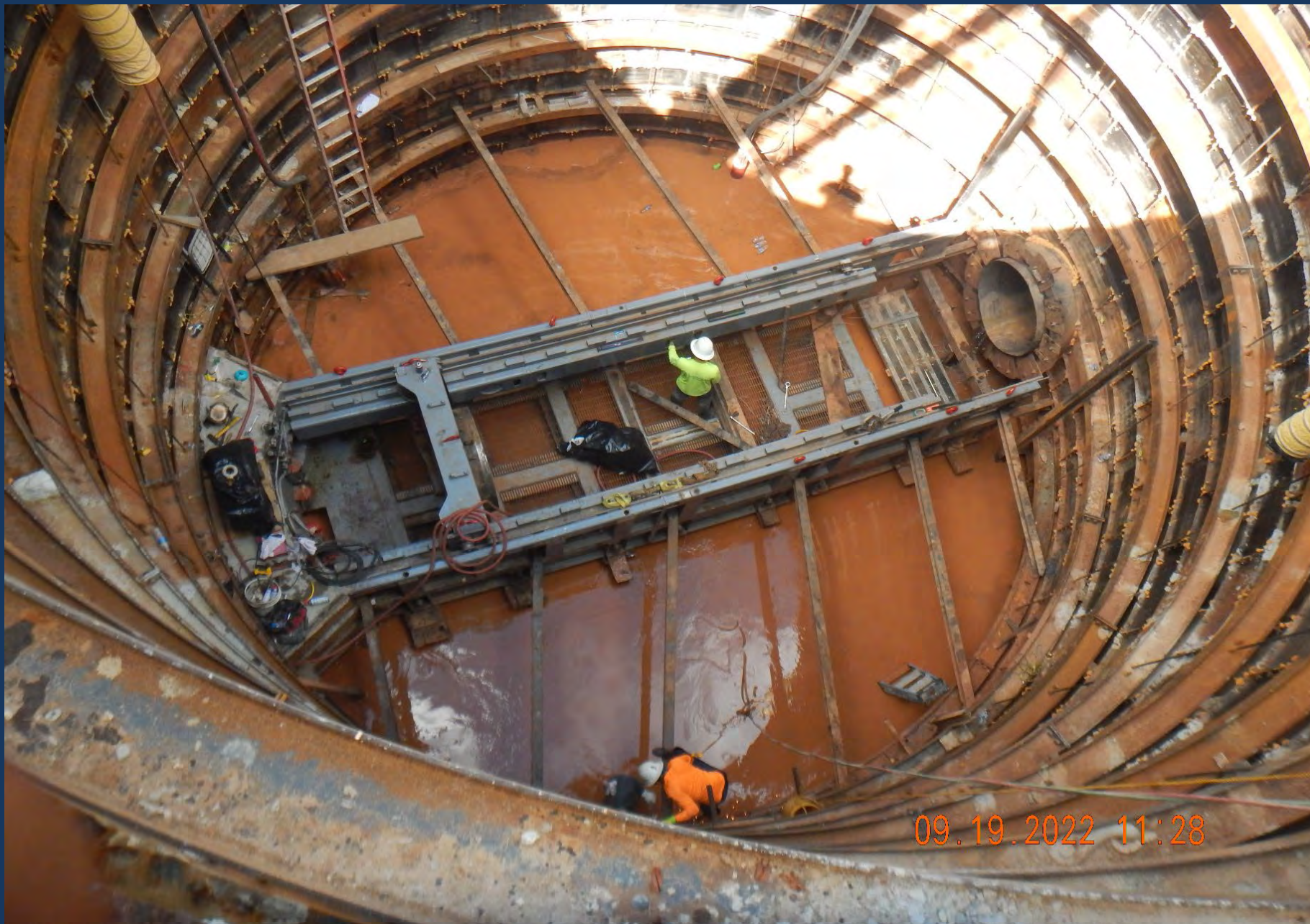
Microtunneling Operation Under Greens Bayou has been completed (Project 25E)
