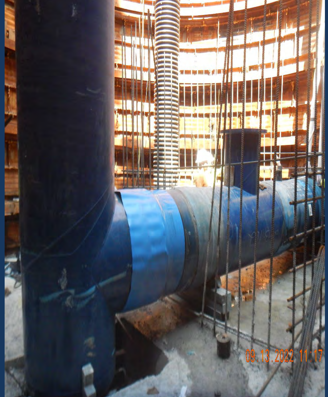
Tunnel threading with 36-inch Steel pipe under HCFC Channel (Project 25E)
