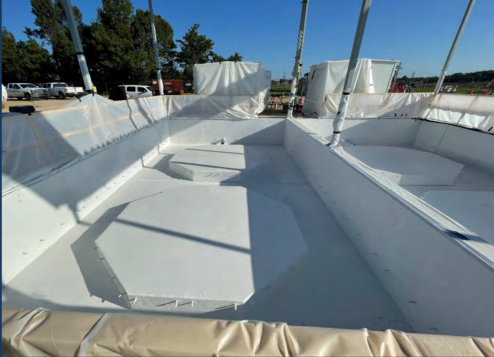
Secondary Containment Epoxy Coating at the new chemical facility
