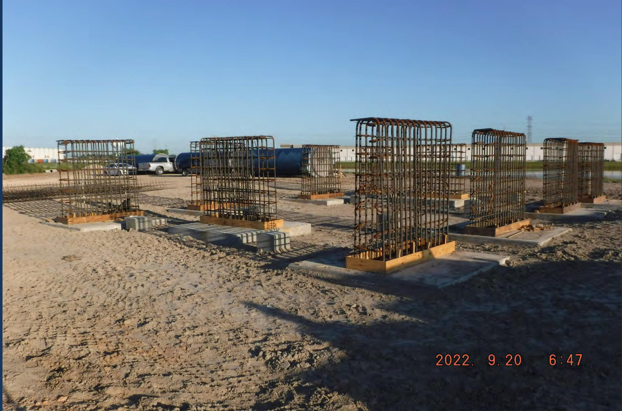
Concrete Thrust Blocks at the new Meter Station Site along Greens Crossing
