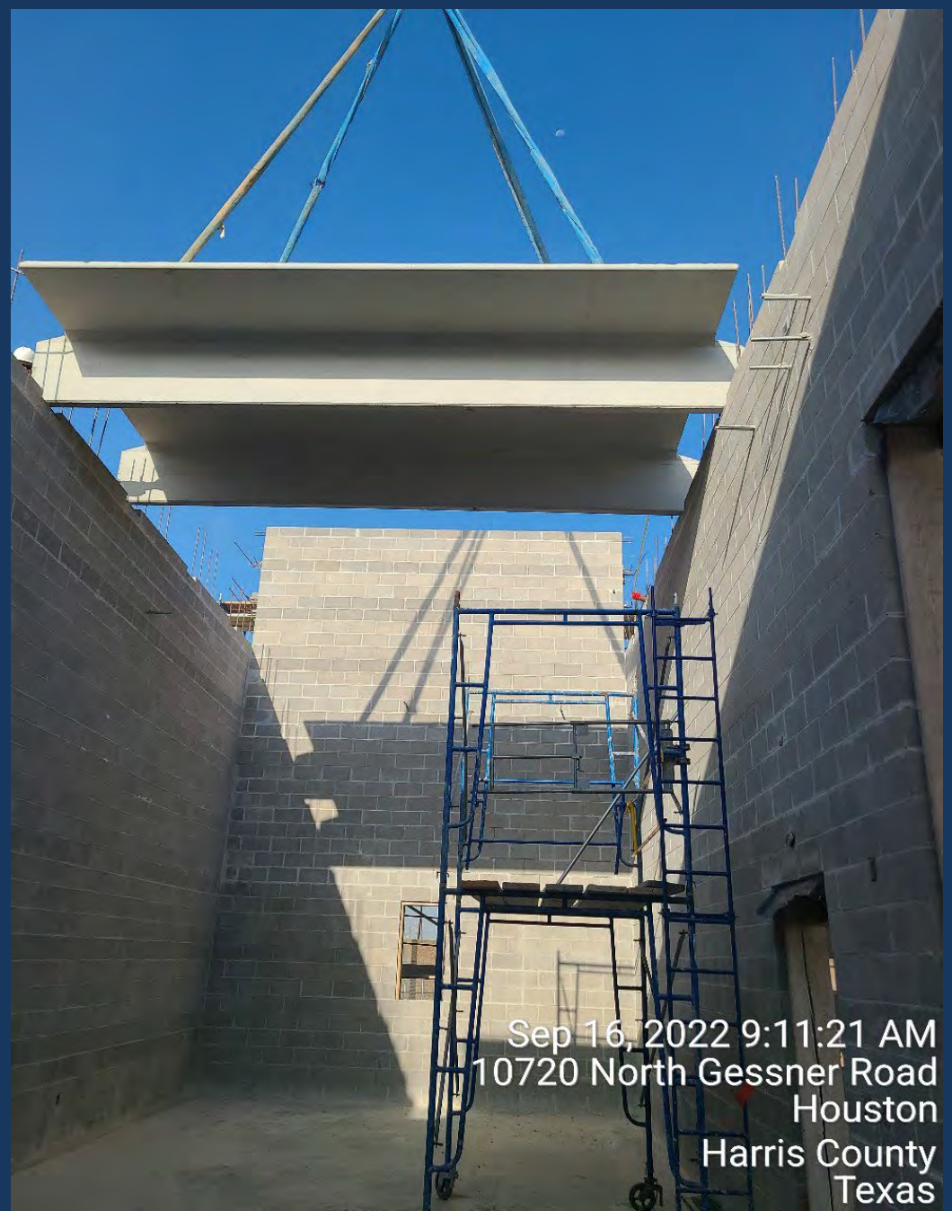
Maintenance Building – Block Walls & double T Beams being set in place
