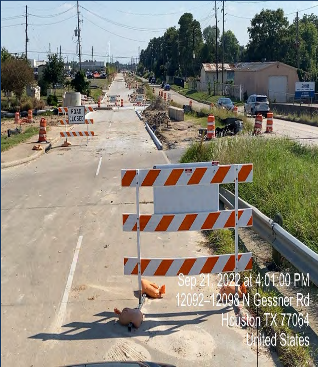
Paving Restoration is on going after Water line installation- NB of Gessner Rd. (Project 28G)
