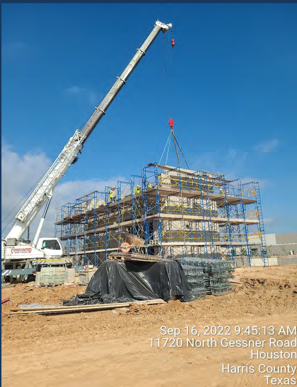
Maintenance Building – Block Walls & double T Beams being set in place
