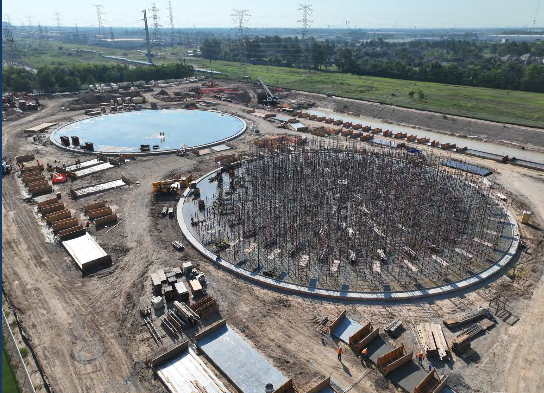
Scaffolding installation at GST #2
