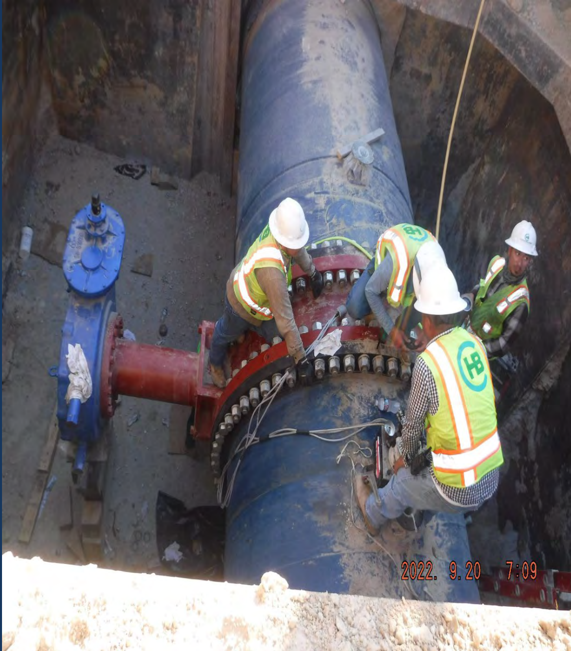
Continue installing 84-inch water Line and Valves via open Cut ( Project 25D)
