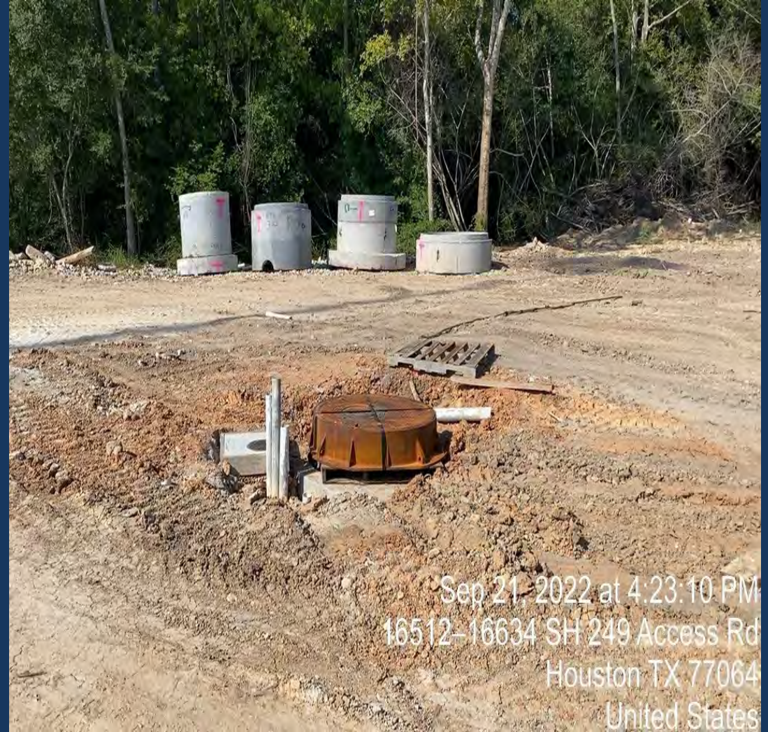
Contractor is performing site restoration, installing manholes, and paving repair (Project 28D)
