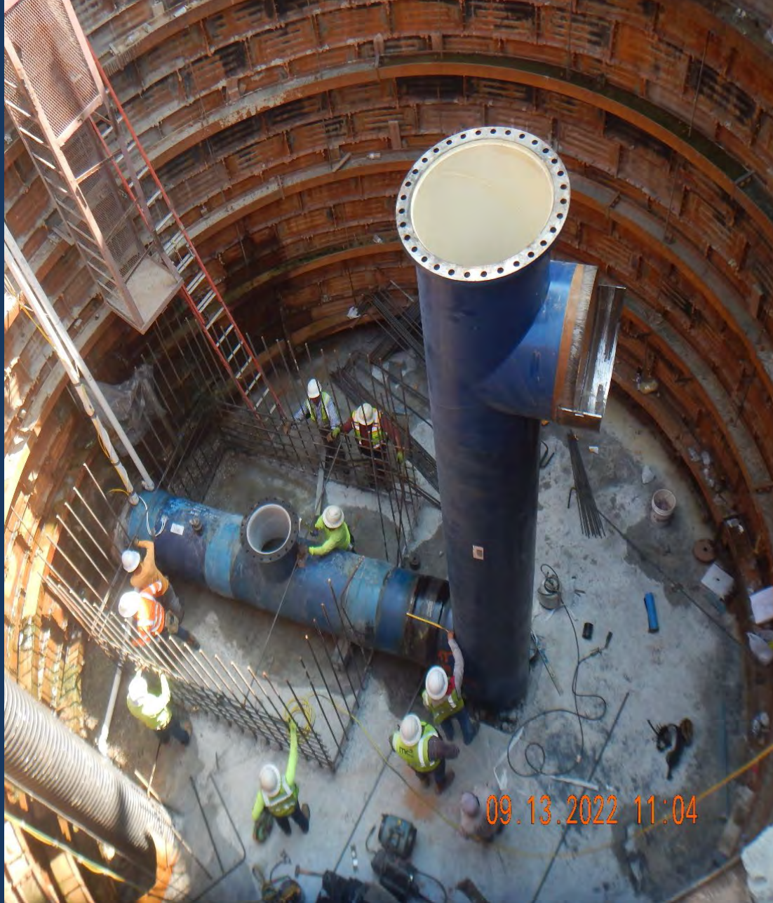
Tunnel threading with 36-inch Steel pipe under HCFC Channel (Project 25E)
