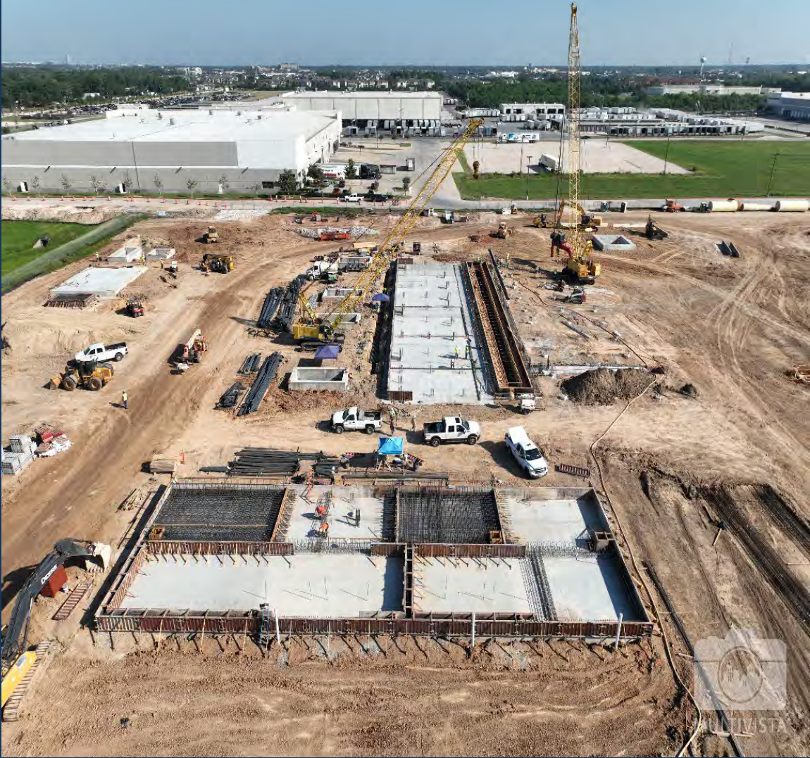
Pump Building – The seal slab for the entire west side of the pump building has been installed
