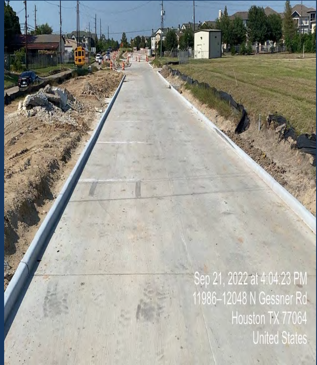
Paving Restoration is on going after Water line installation- NB of Gessner Rd. (Project 28G)
