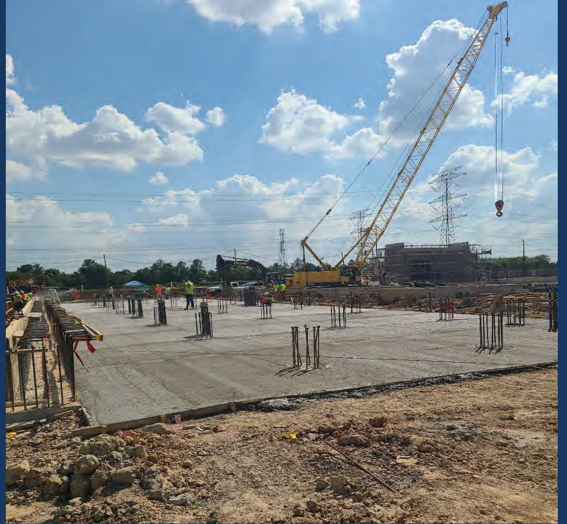
Pump Building – The seal slab for the entire west side of the pump building has been installed
