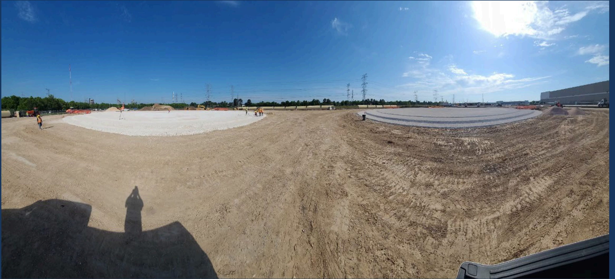
Ground Storage Tank 1 & 2 Pads
