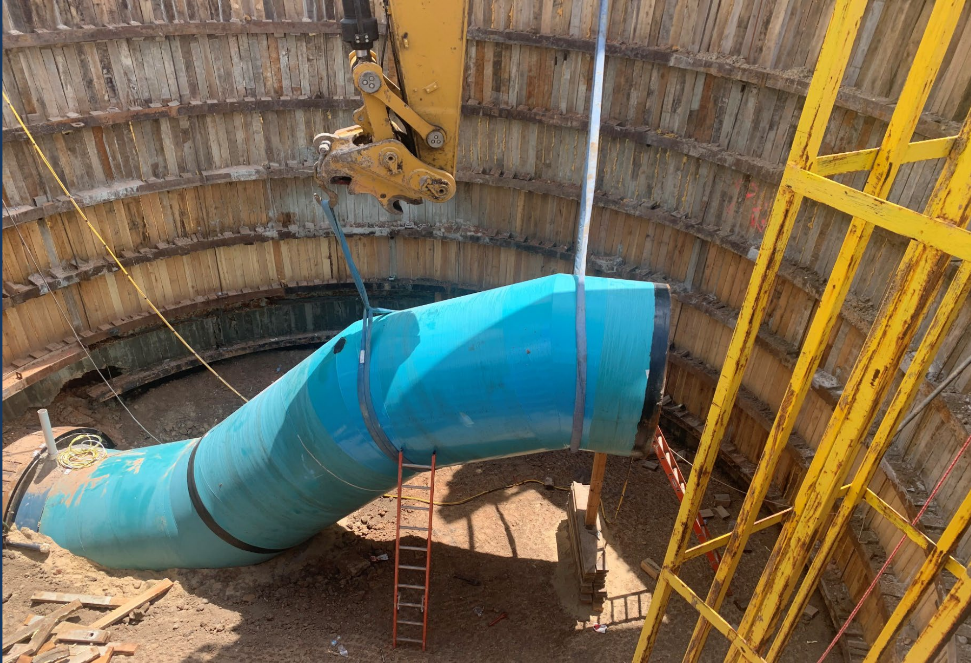
Pipe Fitting installation (Project 28D)
