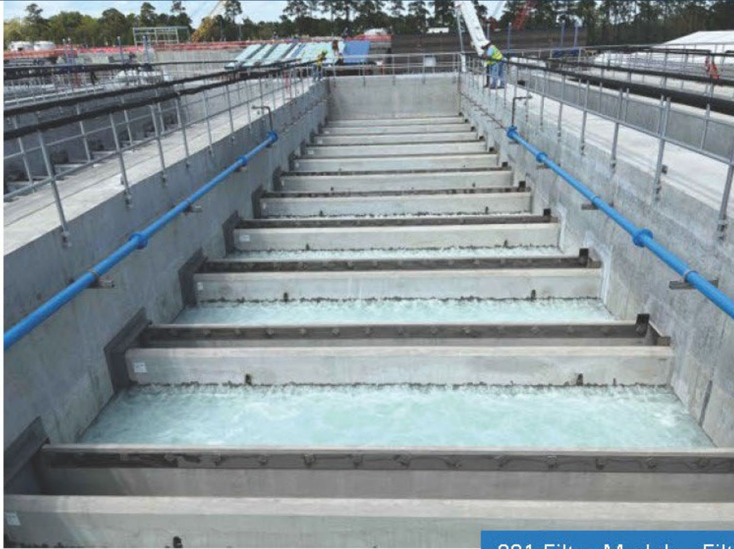
281 Filter Module - Filter UD Testing
