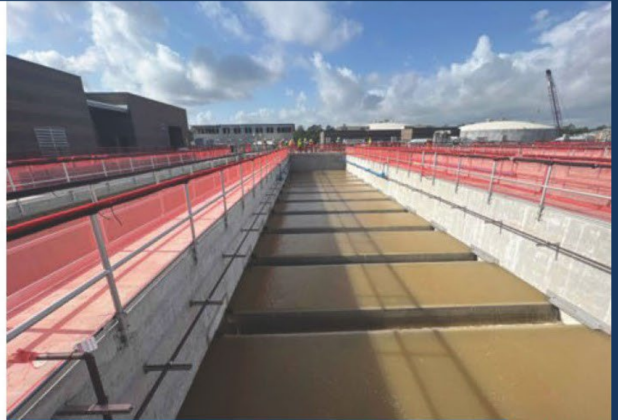
281 Filter Module - Filter Media Backwashing
