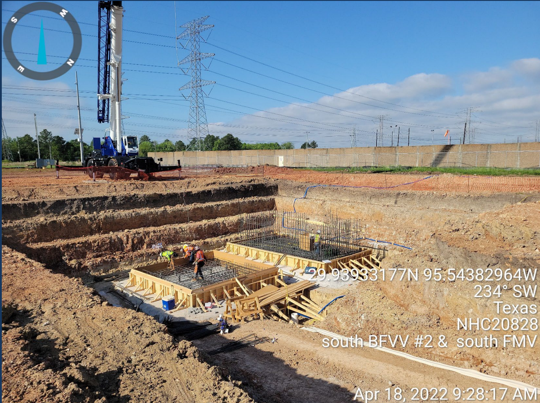
Foundation Forms Installation at the Flow Meter & Butterfly Valve vault
