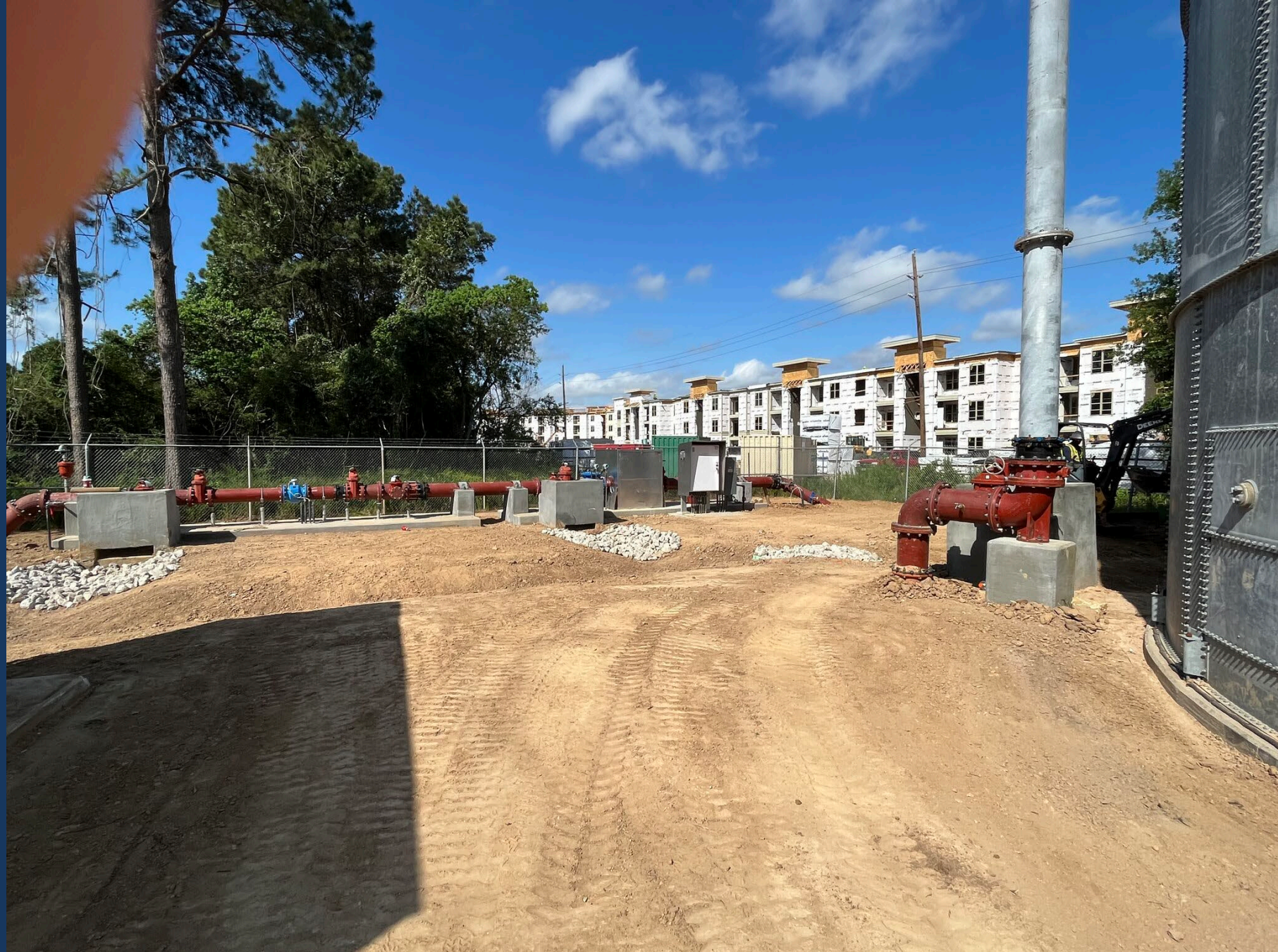
Final Grading and Pipe Coating at MUD 230 Water Receiving Facility
