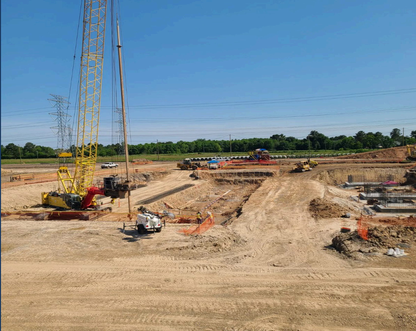
Drill Piers Construction Under the Pump Building
