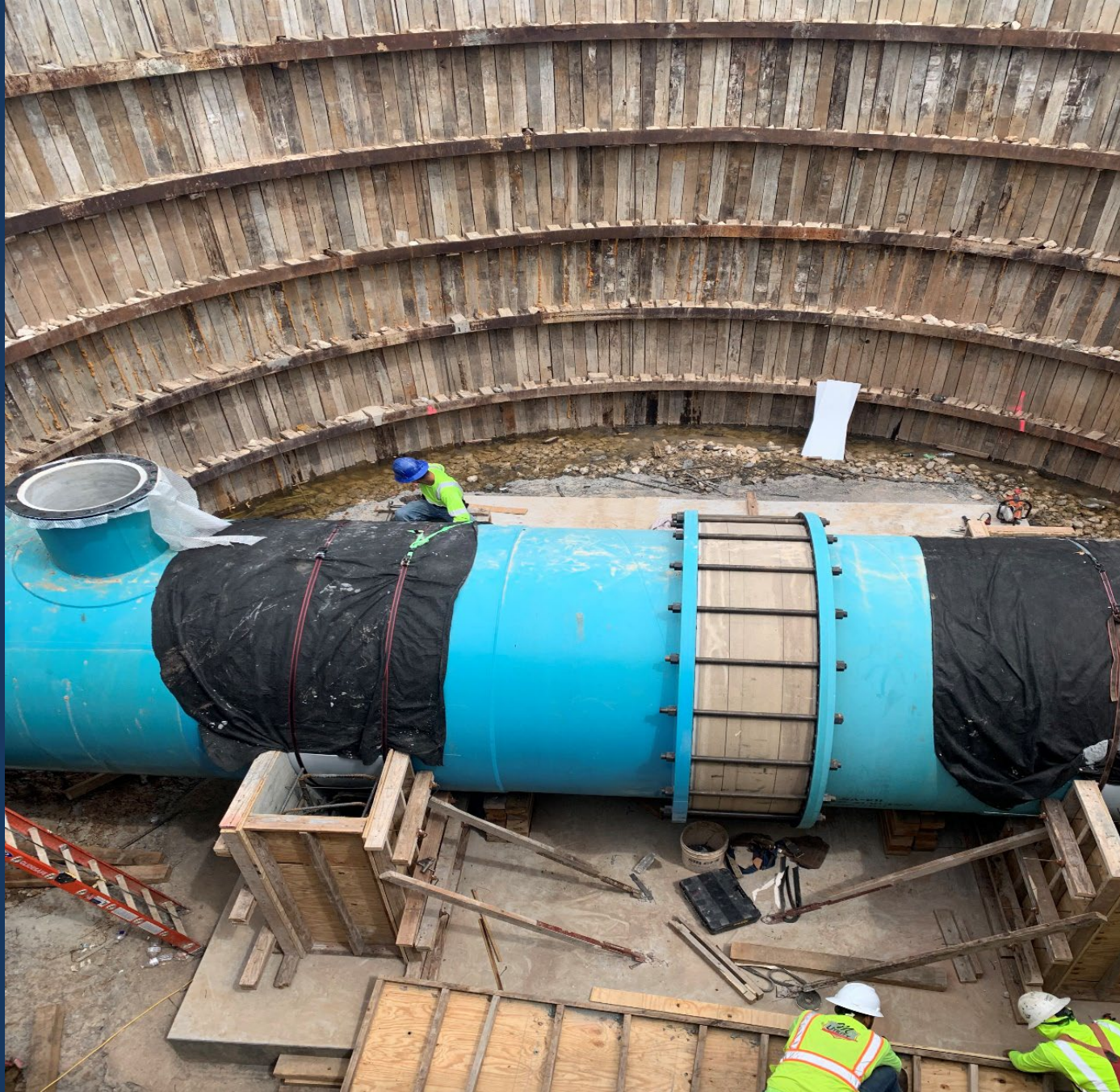
Butterfly Valve Supports Formwork (Project 25B)
