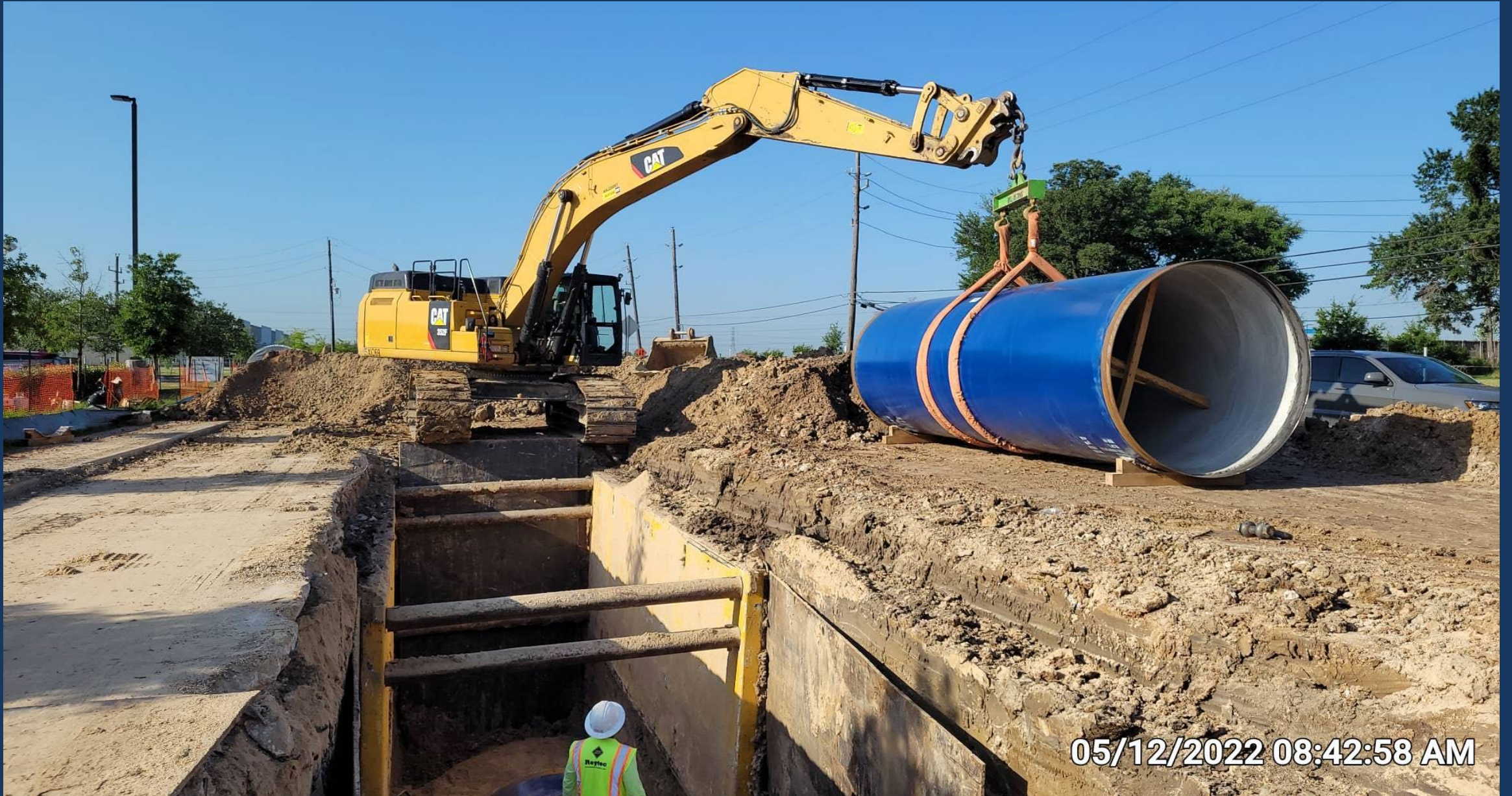
Open Cut Pipe Installation - Under NB of Gessner Rd. (Project 28G)
