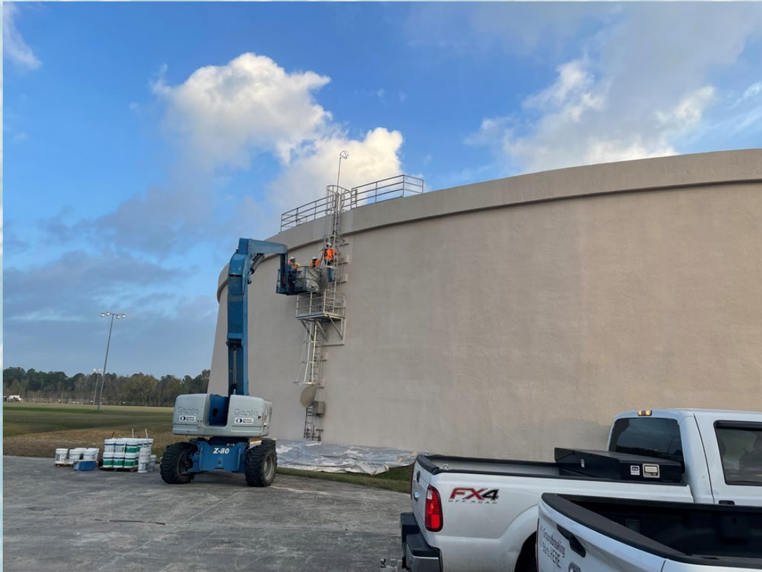
Cleaning and re-coating both Ground Storage Tanks at Spears Rd. Pump Station.
