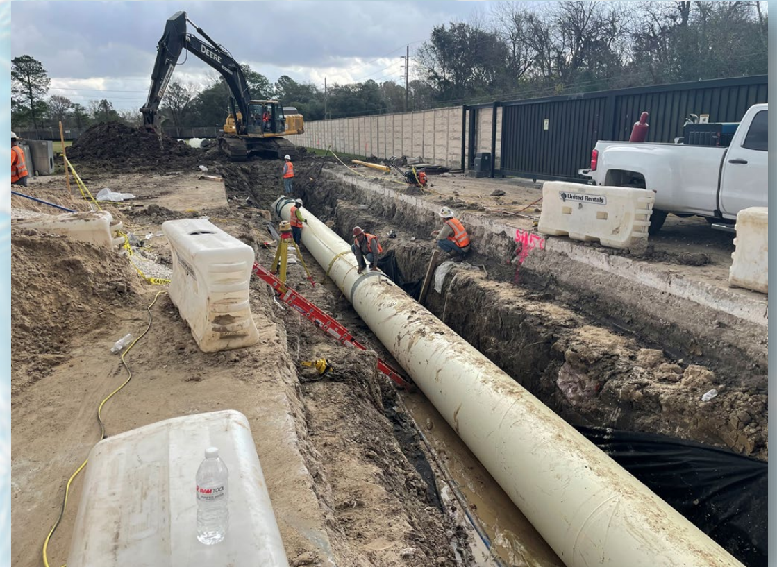
Excavation and installation of 36" steel discharge pipe.
