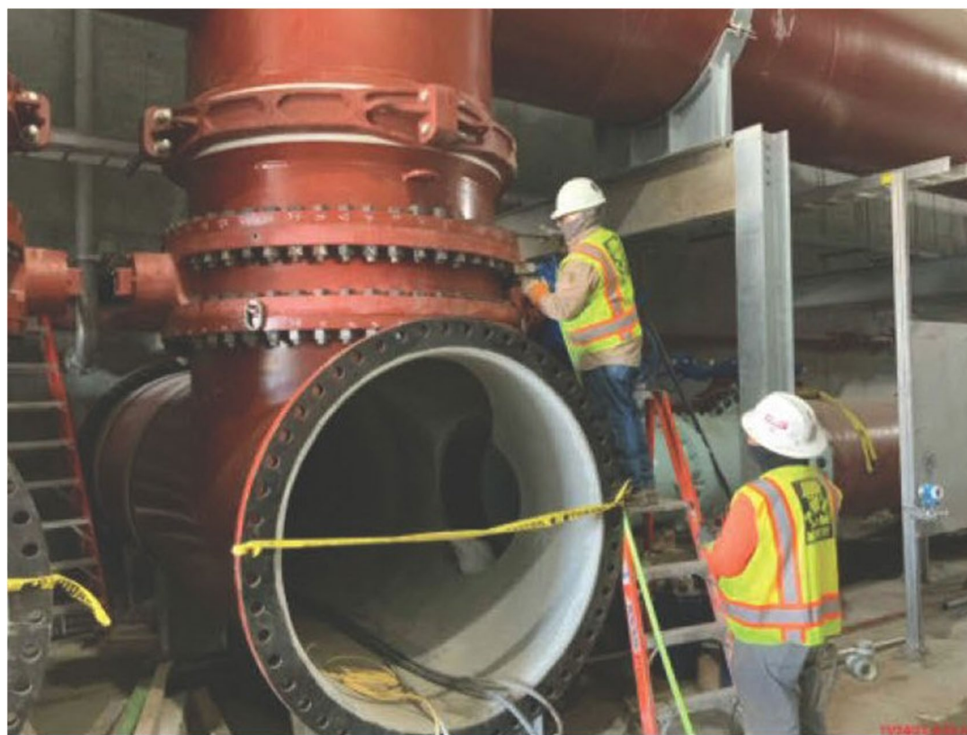
281 Filter Module – Finish Install Large Valves
