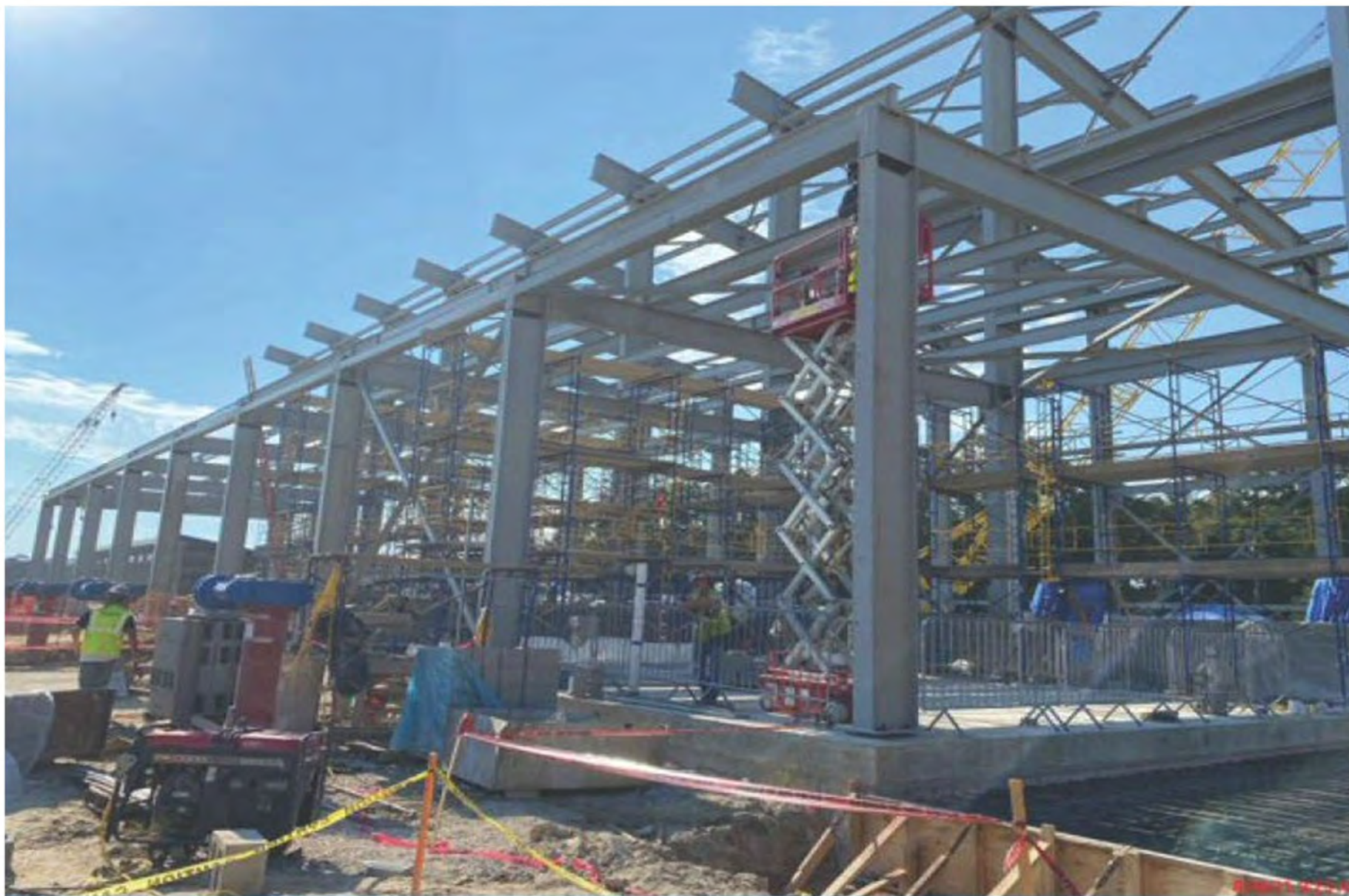
Structural Steel HSPS 401
