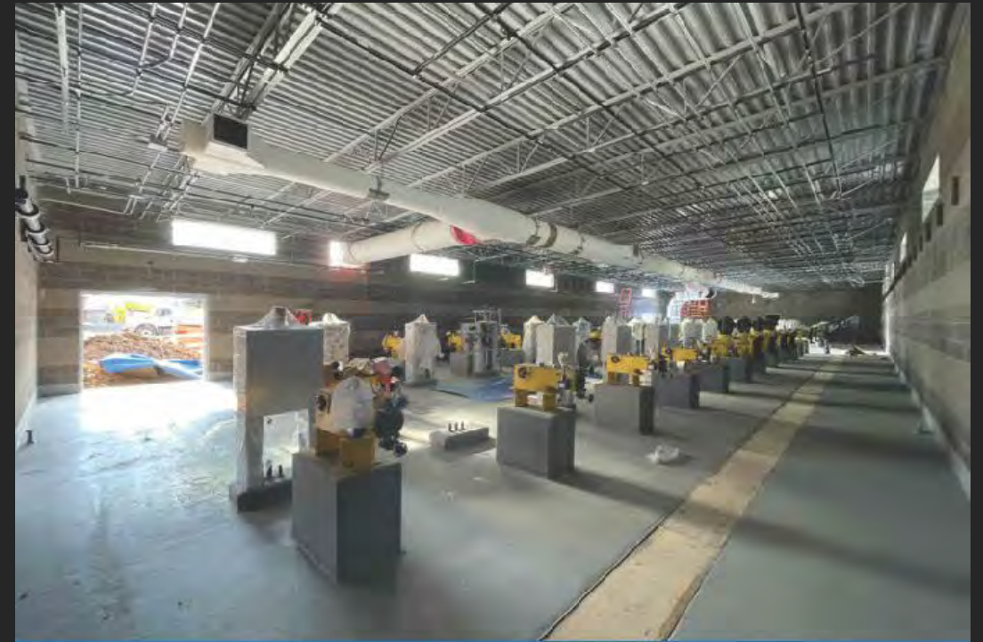
311 – Chemical Metering Pumps Mock-up Installation
