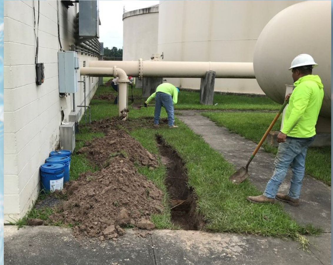
Contractor is digging trenches for chemical lines inside Emerald Forest Plant No.3
