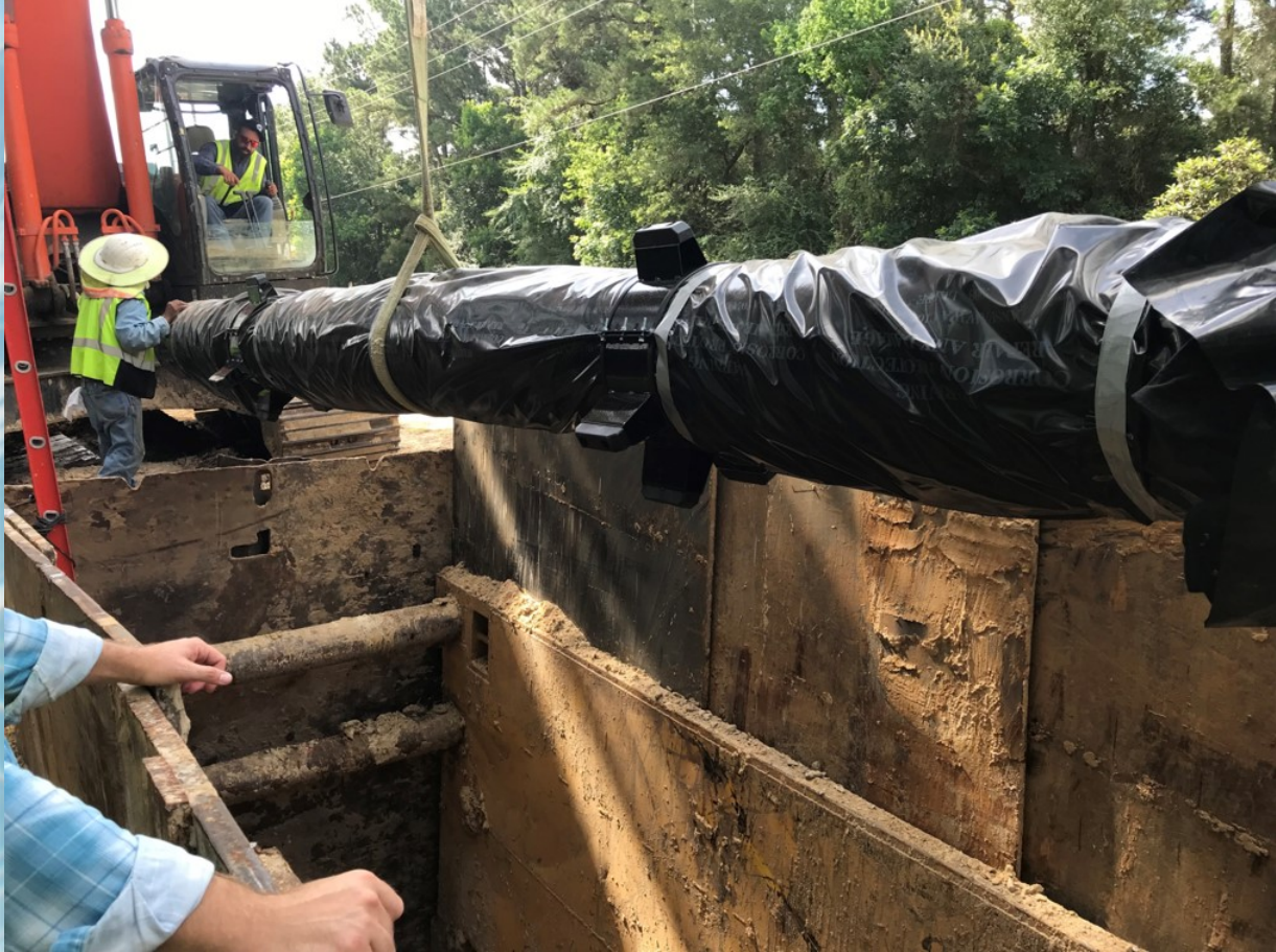
Contractor has started laying pipe and digging bore pits along the first alignment (Along Copeland Dr to Mills Rd MUD No.2)
