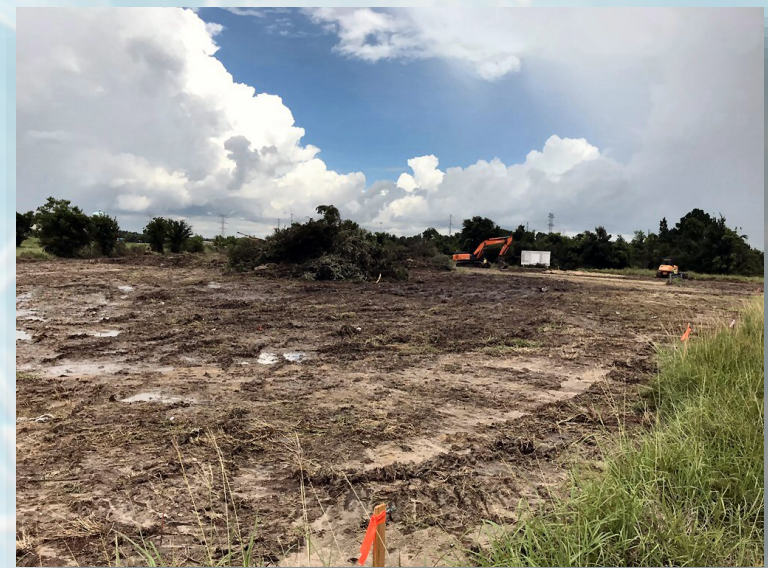
The contractor has completed clearing and grubbing at Meter Station / Pond Site west of I-45
