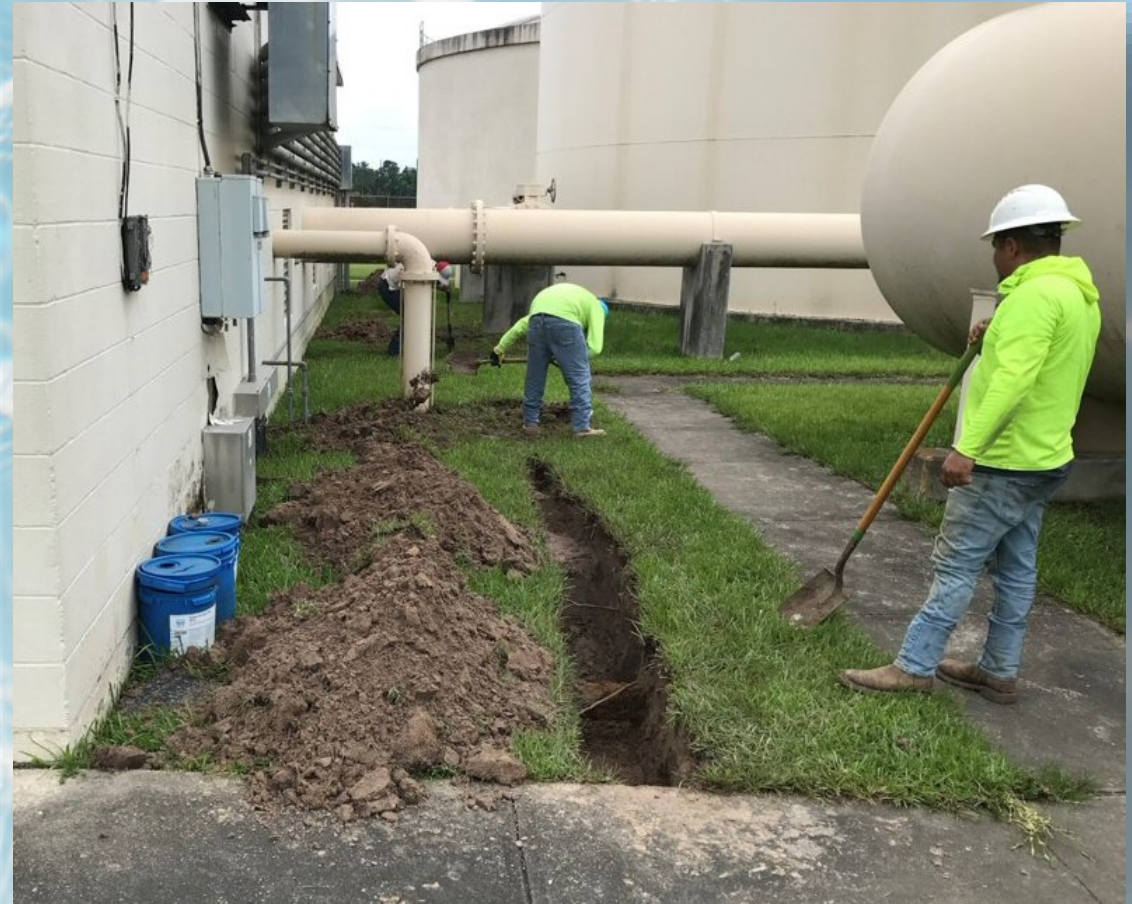
Contractor is digging trenches for chemical lines inside Emerald Forest Plant No.3
