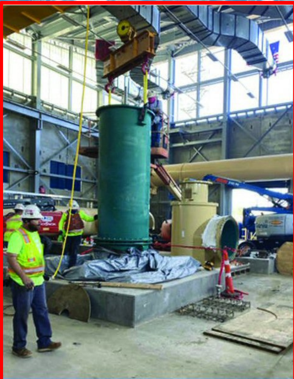
VT Pump Install at IPS
