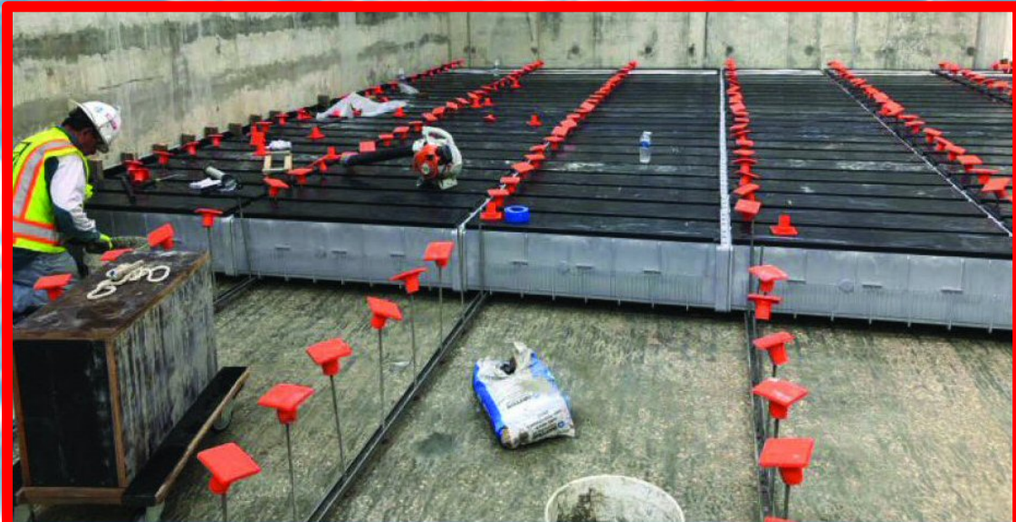
Underdrain Install – Facility 281 Filters
