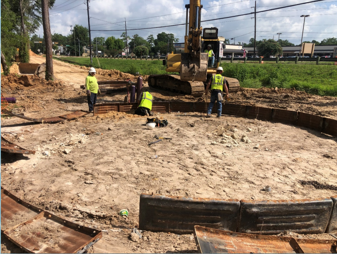
Dismantling the launching shafts has been started.
