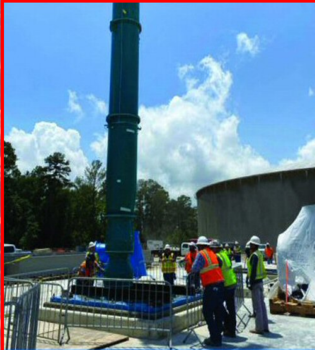
Install VT Pump Facility 401 HSPS
