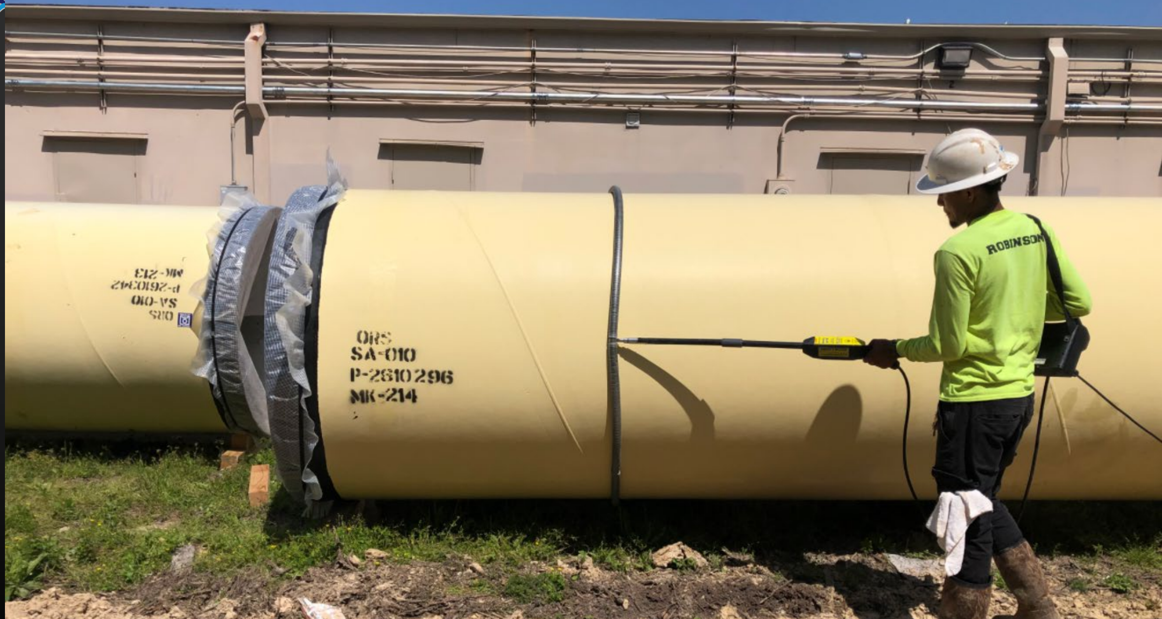
Holiday Testing of Pipe Coating on 54-inch
