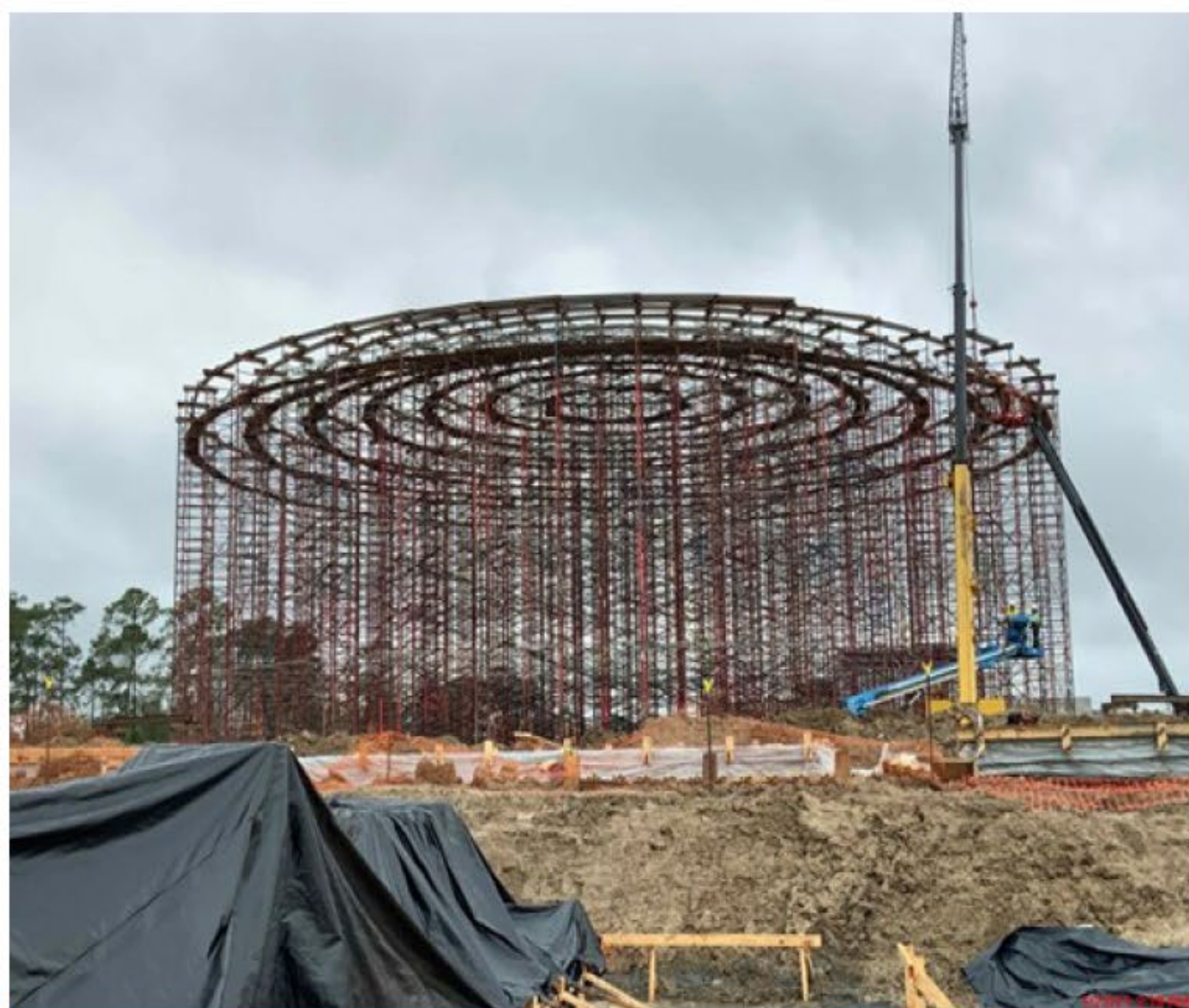
Continued Dome Shoring Erection at Facility 362 GST
