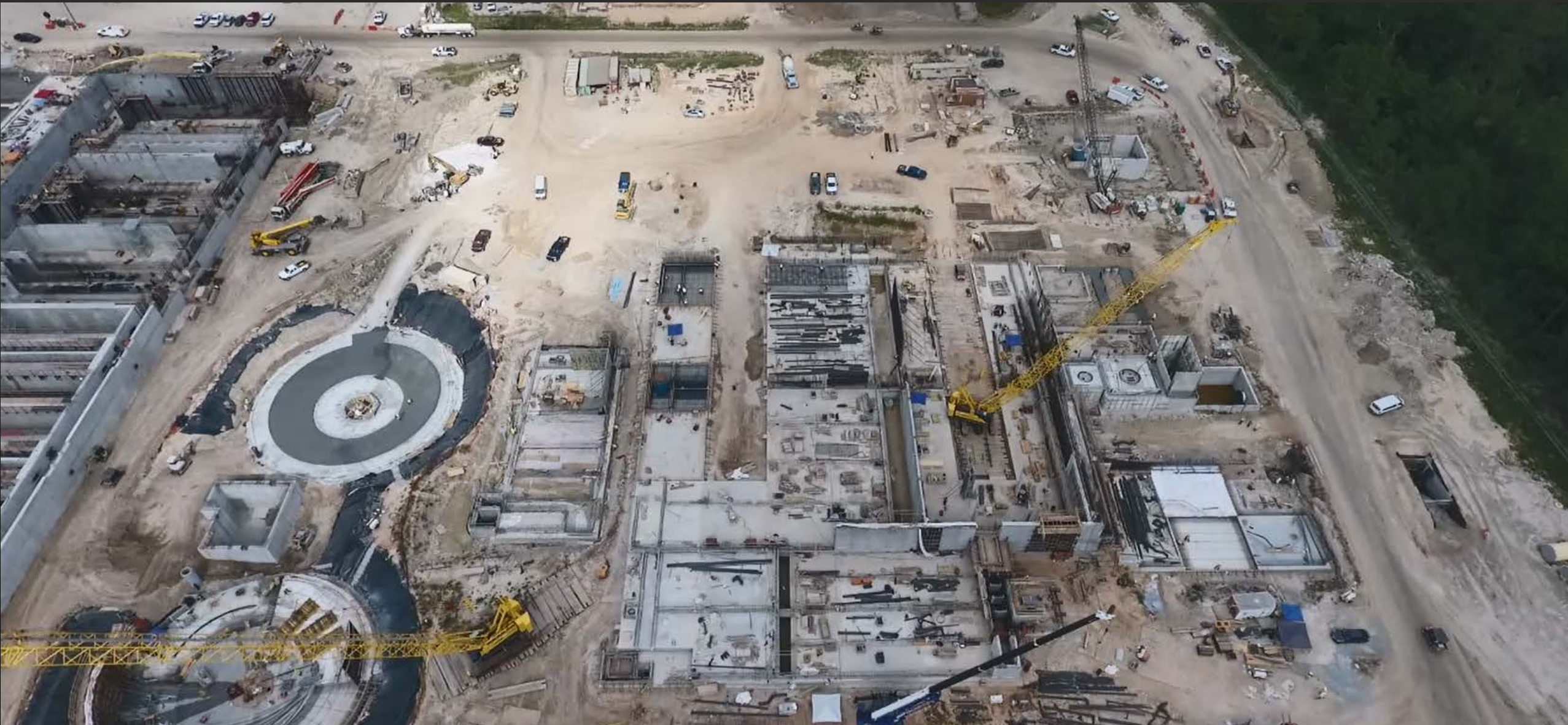
NEWPP Expansion Project
