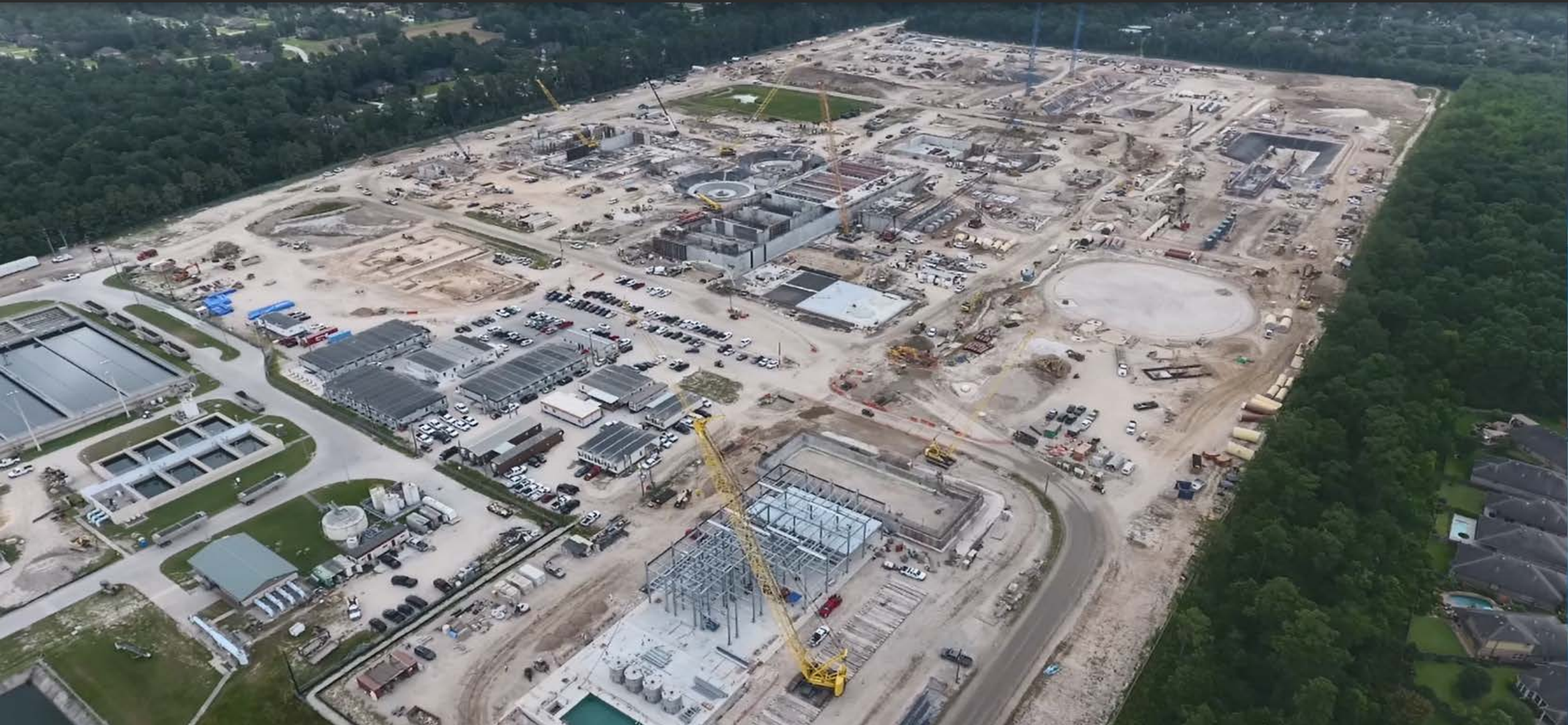
NEWPP Expansion Project
