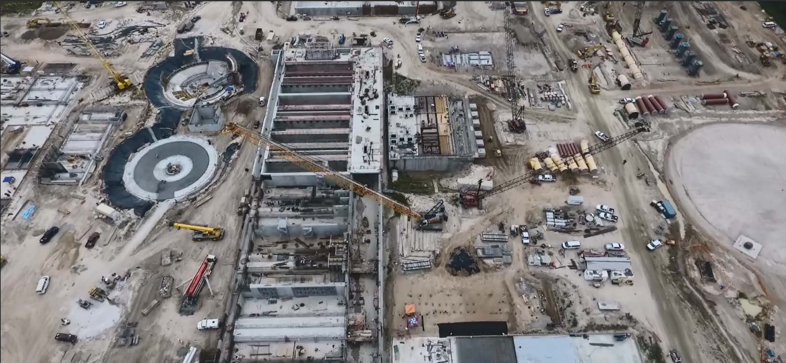
NEWPP Expansion Project
