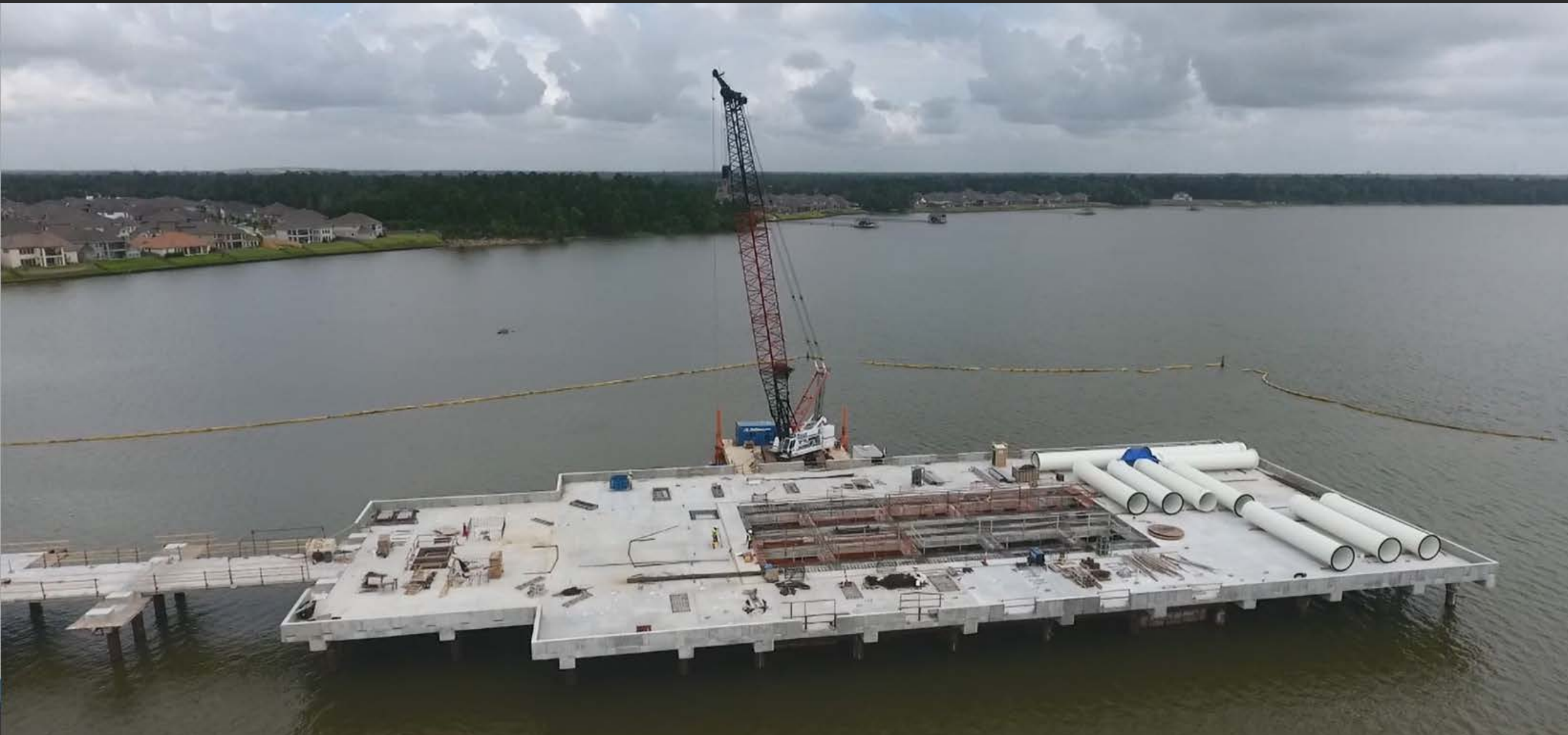
Lake Houston Intake Pump Station
