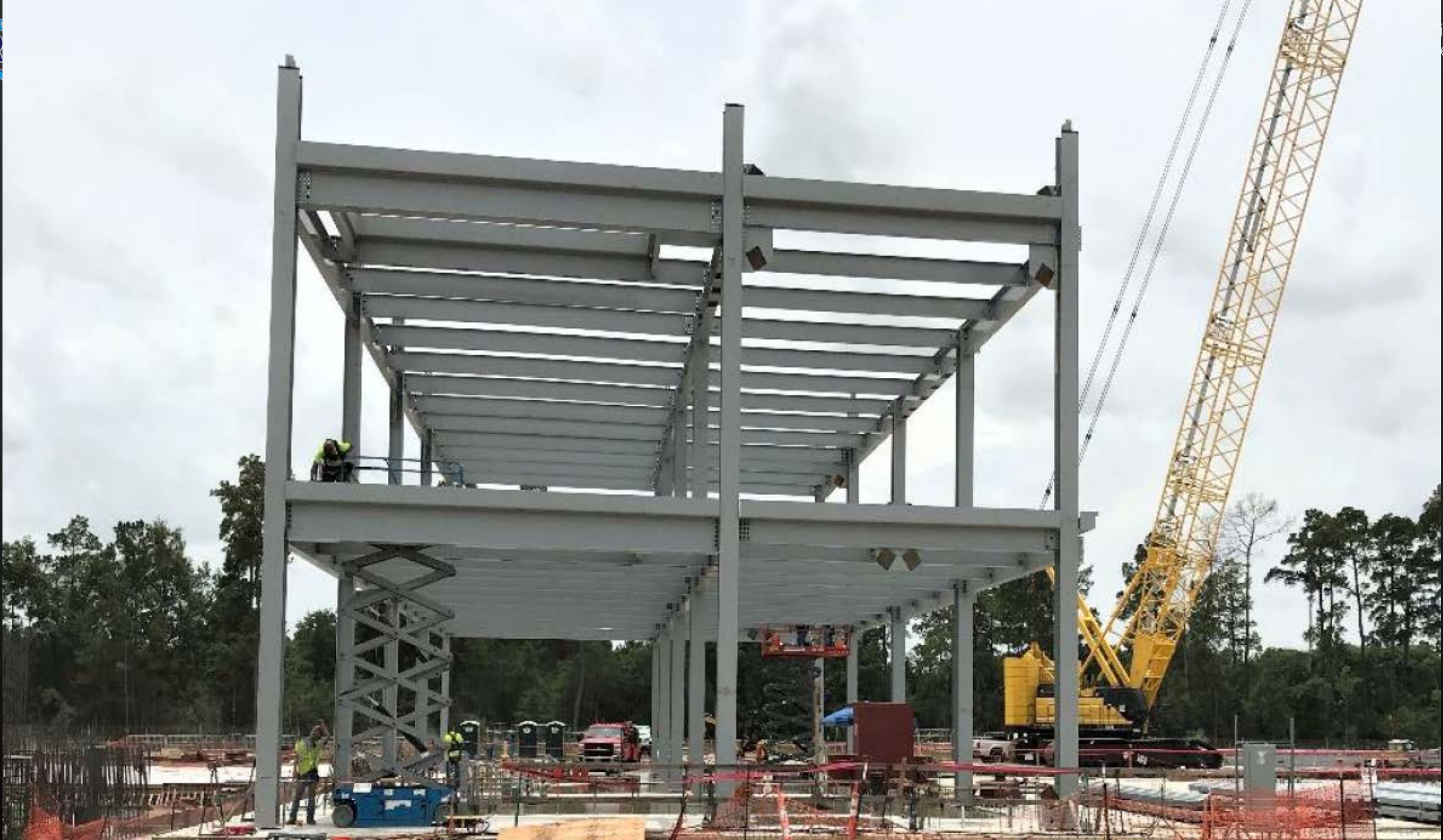
Dewatering Building – Steel Framing
