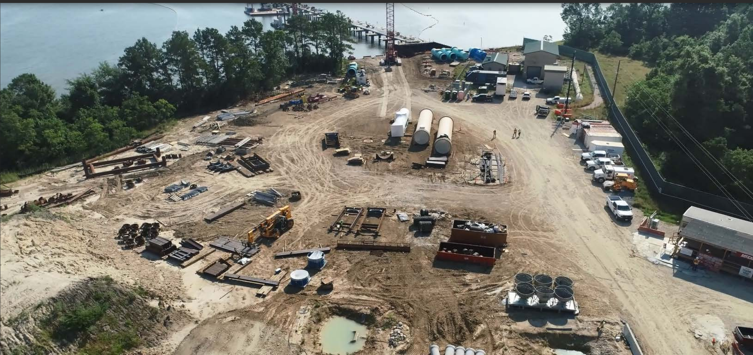
Existing & New Raw Water Facilities at Lake Houston
