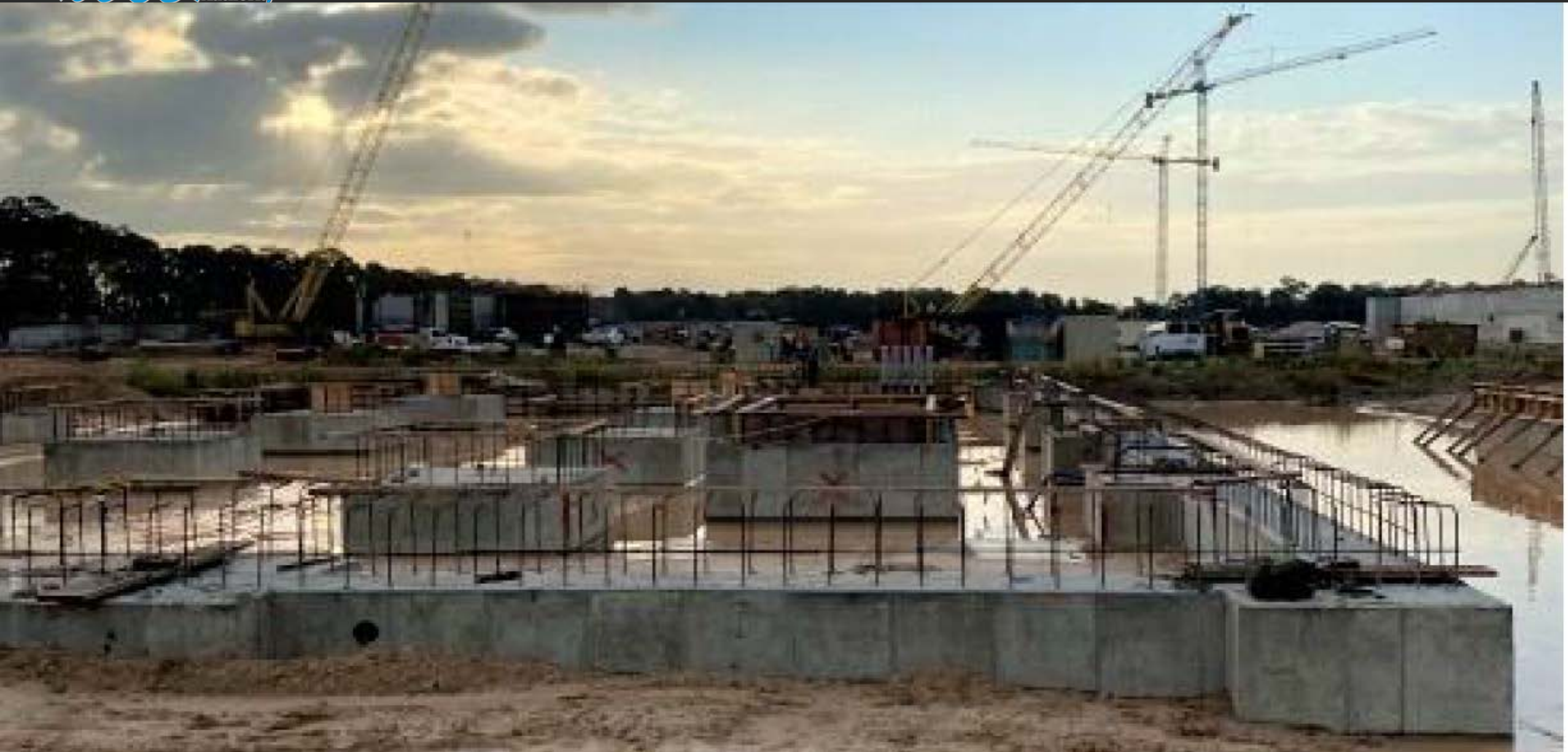
Administration Building – Foundation
