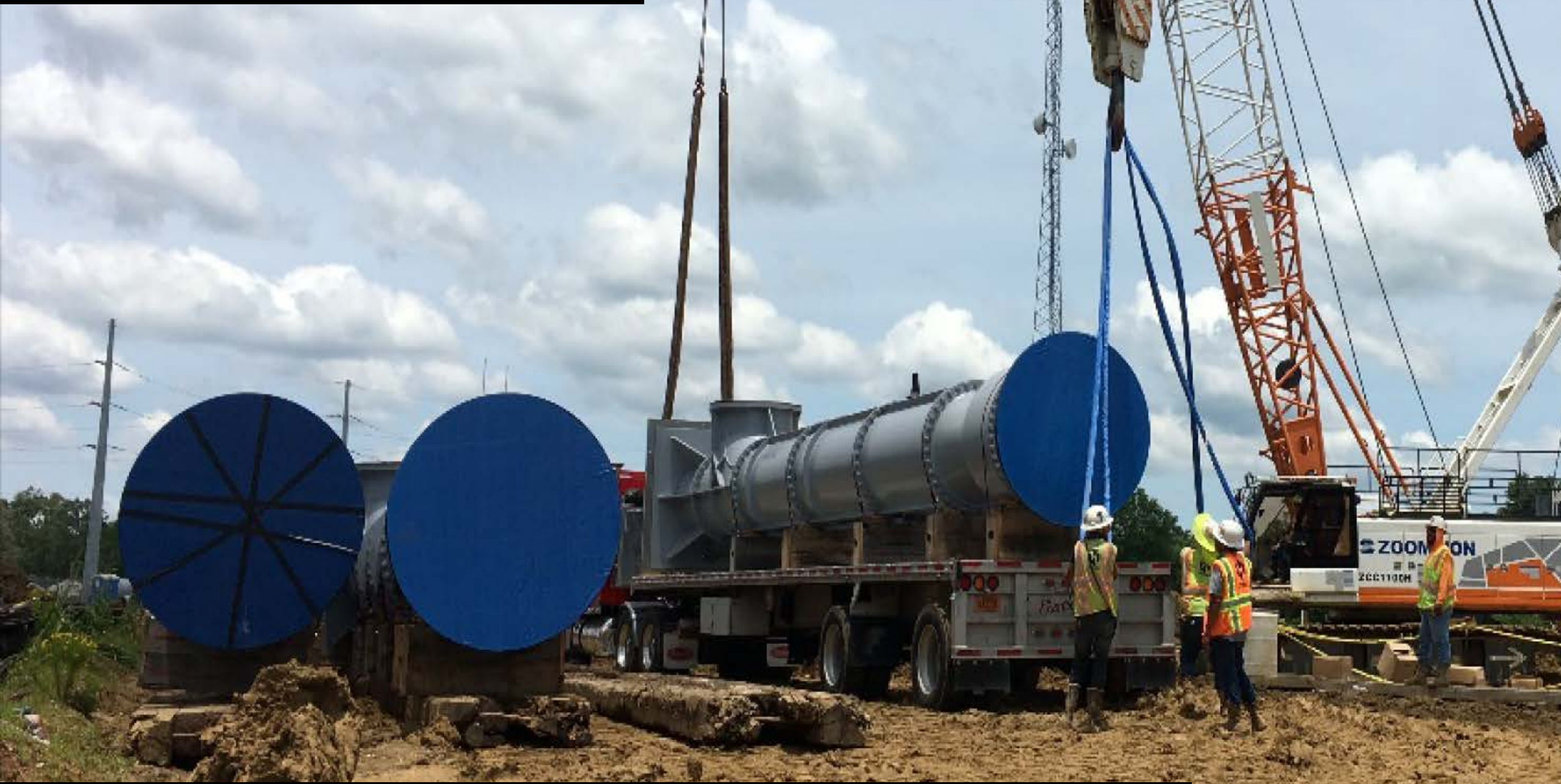
Vertical Turbine Pump Cans - Capers Ridge Pumping Station – Trinity River
