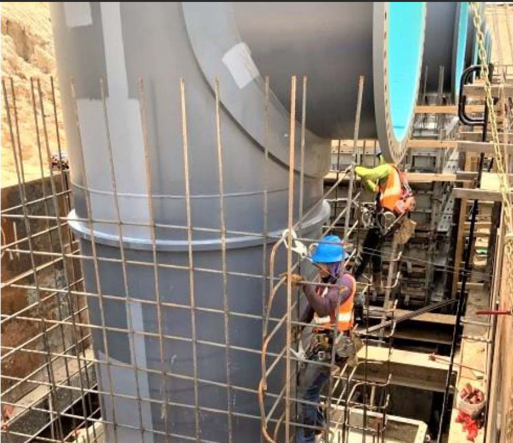
High Service Pump Station – 7 Vertical Turbine Pump Cans
