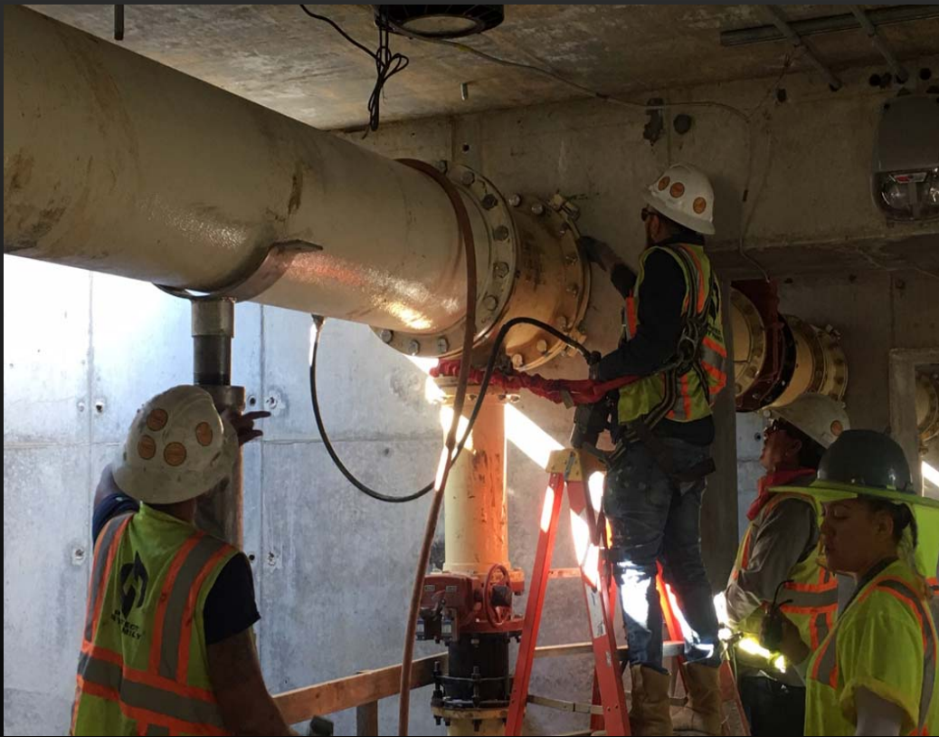
9-inch & 18-inch Flushing Piping
