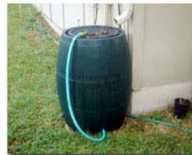
Plastic barrels are becoming a fixture at more and more Austin households, thanks to the city's promotion of rainwater harvesting. Rainwater captured from the roof is used to irrigate a homeowner's lawn and garden. / Photo by city of Austin
